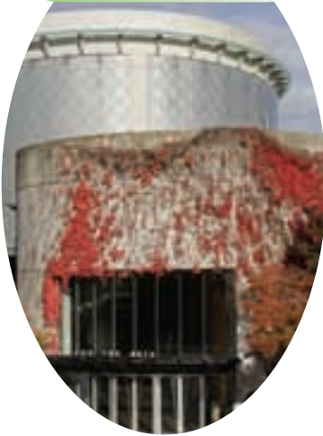
Chan Centre, Vancouver
