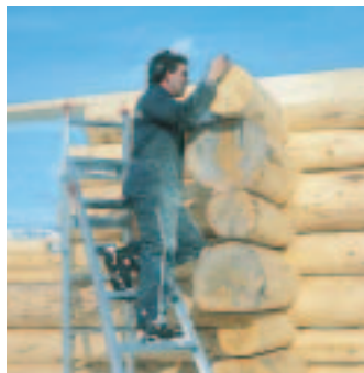
Figure 3.9 The notches cut into these logs ensure that the parts in this structure will remain tightly interlocked. Furniture uses notches for strong joints.
