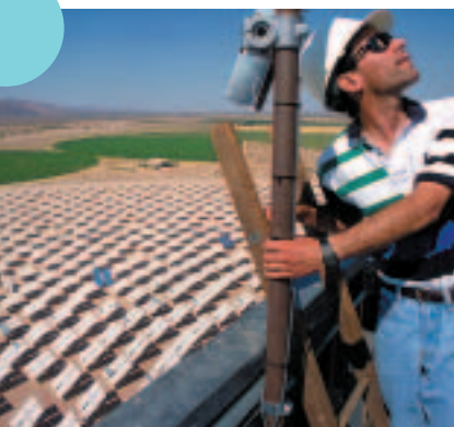
Figure 3.8 This photo shows a different kind of solar array. Here, an array of hundreds of mirrors reflect solar energy onto a water-filled tower. This heats up the water to produce steam, which is used to generate electricity. Such arrays are set up in desert areas where there is plenty of sunshine and little rain.
