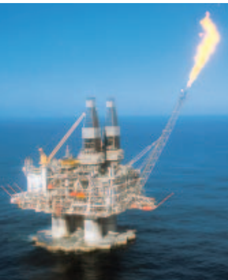
Figure 4.3 Special technology is needed to drill below the ocean floor and to transport the oil and natural gas to shore.
