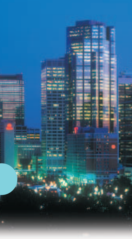
Figure 4.12 Leaving lights on in empty offices overnight wastes electricity.
